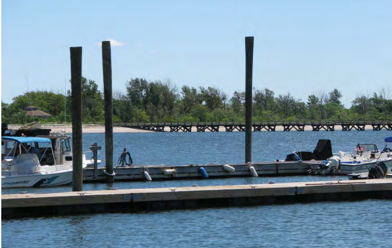
View toward Pleasure Beach from East End | Source: Stantec
