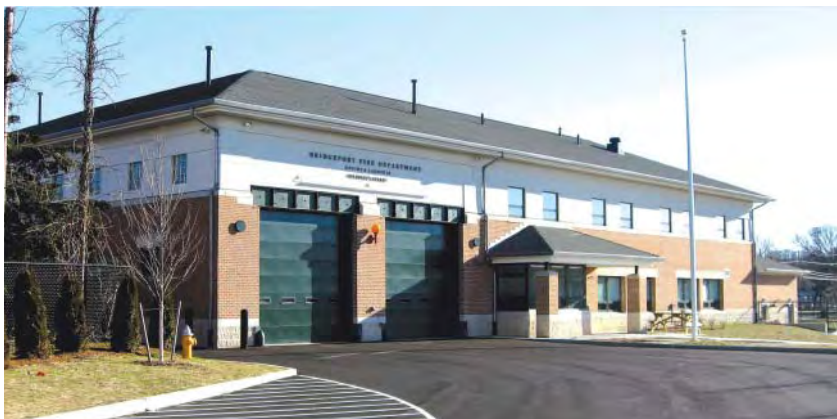
Newly constructed firehouse on Boston Avenue | Source: City of Bridgeport Fire Department
