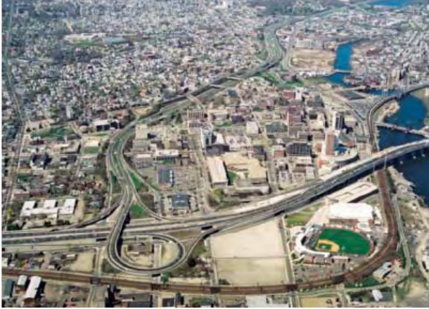
Aerial view of Downtown Bridgeport showing key infrastructure elements: I-95, Routes 8/25 and Metro-North railroad. Source: Phillips Preiss Shapiro Associates
