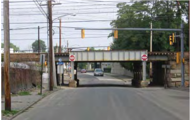
New Haven Rail Line | Source: Stantec
