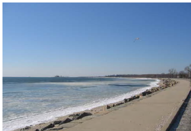
Seaside Park Shoreline | Source: BFJ Planning, 2007
