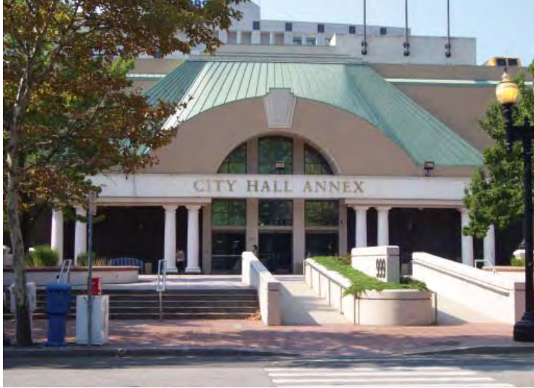
City Hall Annex, 999 Broad Street Source: BFJ Planning
