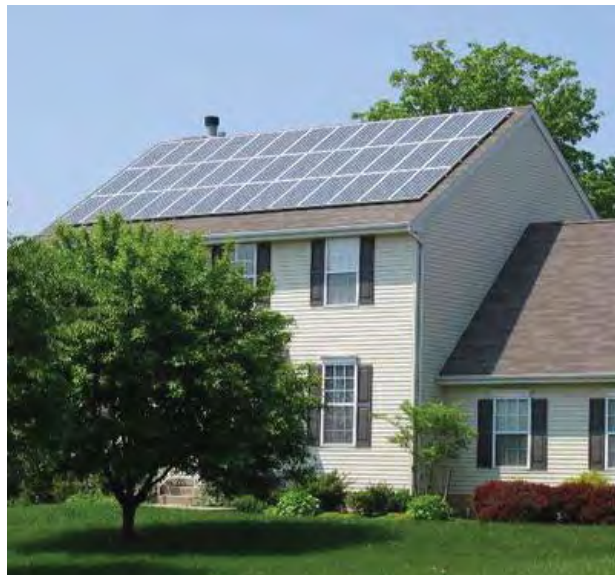
Roof-mounted solar panels | Source: Stantec
