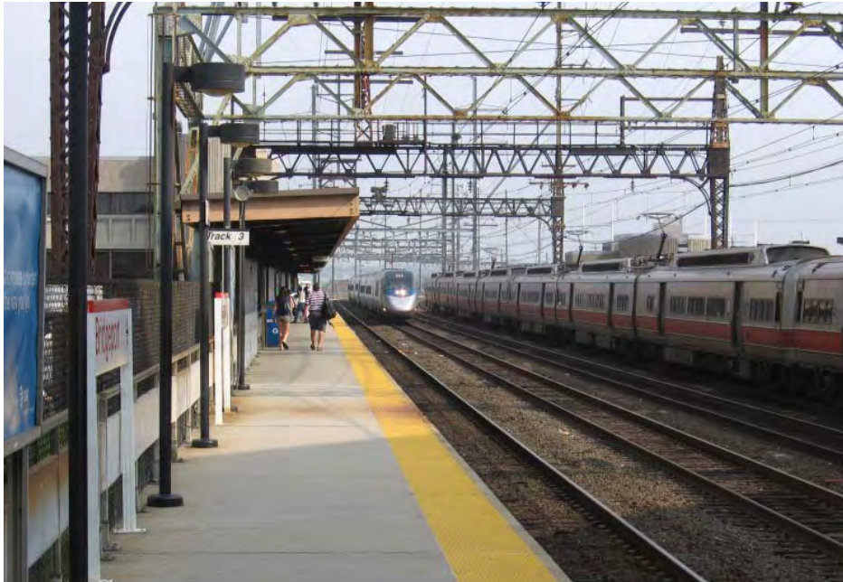
Metro-North Railroad Source: Stantec
