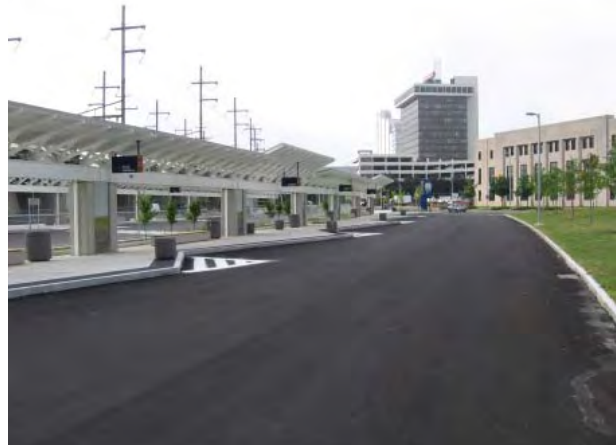
Inter-modal Center (front view) | Source: Stantec
